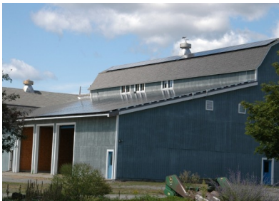
In 2009, our photo-voltaic system generated over 67,000 kilowatt hours of electricity.
